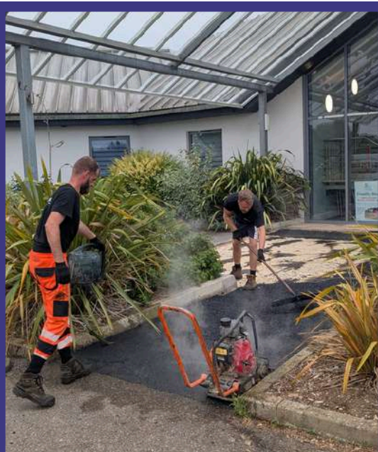
We are hugely grateful to Kent Construction Consultants who organised to replace our tiles with fresh tarmac and make our entrance safer for all.
